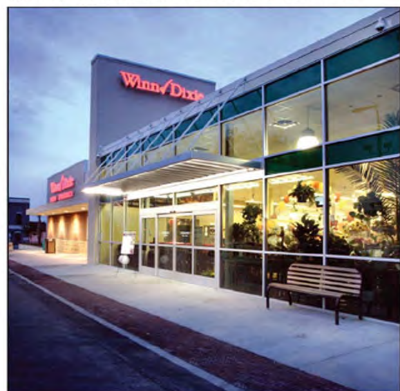
■ Store #37 is the only full-service grocery store serving downtown Jacksonville. The contemporary store front was designed to reflect the urban architecture of the area.
