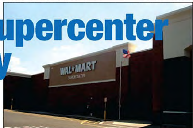
■ WAL-MART opened a new Supercenter outside of Garner, N.C., July 16, replacing a smaller store while continuing its 18-year commitment to the community.
