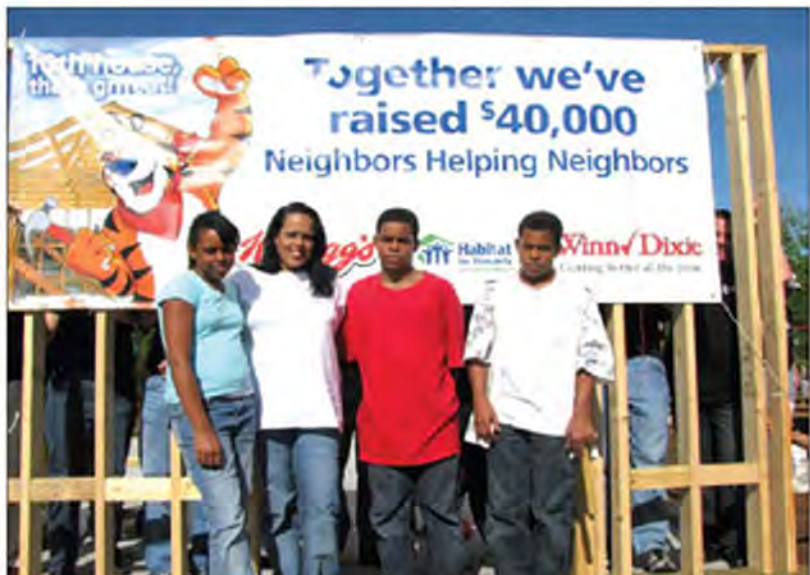
■ Sandra Pastrana (second from left) and her children (left to right) Kasha, Carlos and Juan, raised the first wall of their future Habitat for Humanity home with the guidance of Habitat.
