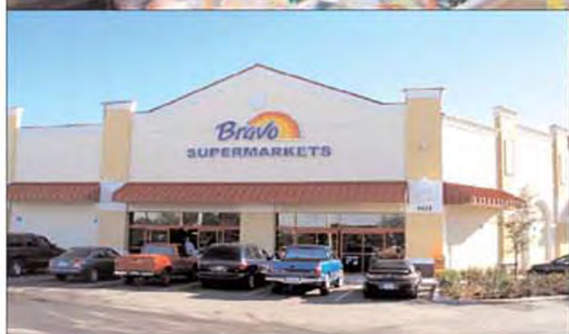
■ BRAVO SUPERMARKET opened this showplace supermarket formally on December 6. The new store — at 15,000 sq. ft. — may not be the largest for the company in Florida, but certainly represents one of its most unique and appealing. The store is located at 4651 Old Pleasant Hill Road in Poinciana near Kissimmee.
