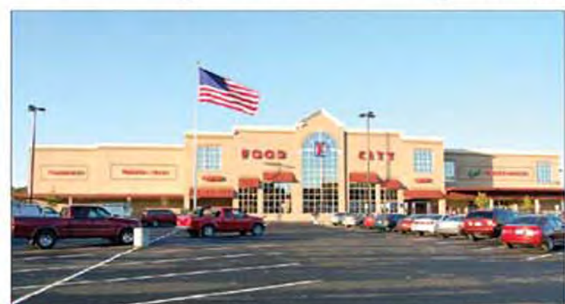
■ The new Eastman Road Food City, which opened November 14, replaces an earlier store which was demolished to make room for the new project.
