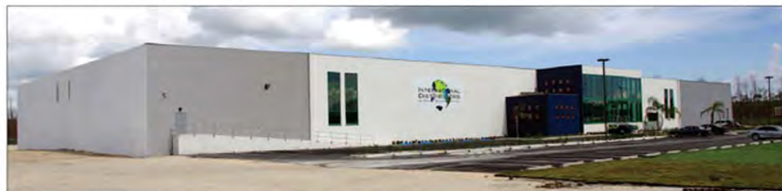
■ CONSTRUCTION COMPLETED — Work has been completed on Phase 1 of IDGBL's new home in Freeport, Grand Bahama. A formal grand opening ceremony for the new facility is scheduled for later this month.
