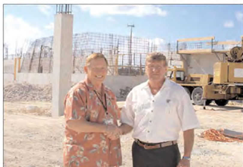
■ Standing inside the job site with their backs to what will be the IDGBL corporate offices, are IDGBL President Roy Deffler and AG of Florida President/CEO Cal Miller.
